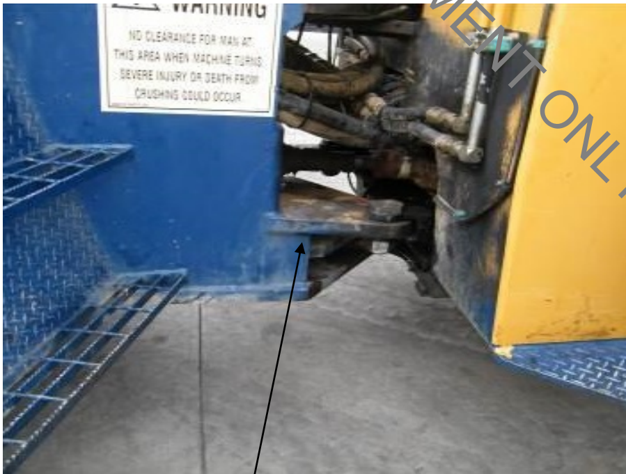
New articulation pins and bushes replaced.
